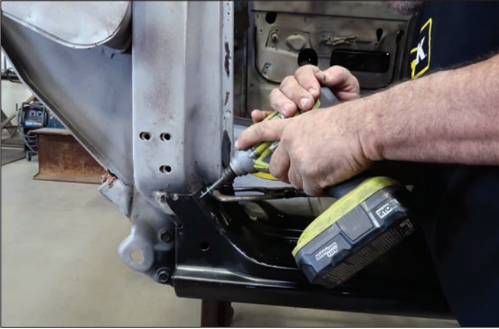
3 After pre-drilling some holes and spraying some weld-through primer on the inner panel, Mike temporarily screws the outer replacement panel to the body.
